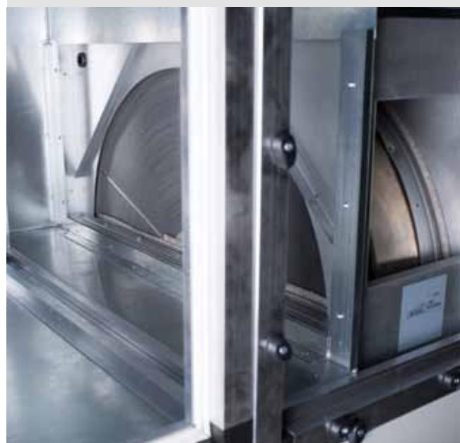
To ensure a better efficiency and different AHU modes according to the requirements and ambient conditions (defrost, free cooling and recirculation), the heat recovery exchangers are equipped with bypass and recirculation dampers.
